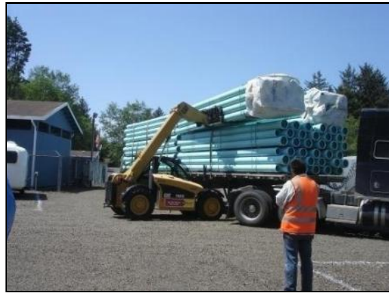
Larry Hampton watches unloading of water line pipes.
