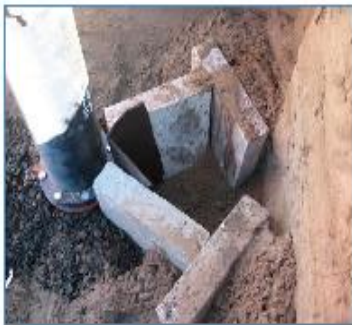
Fire Hydrant Ready for Thrust Protection
