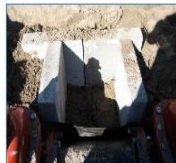
Hydrant Tee Ready for Thrust Protection
