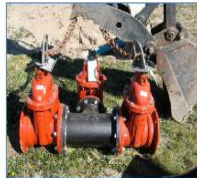
Valves are Flanged for Thrust Protection
