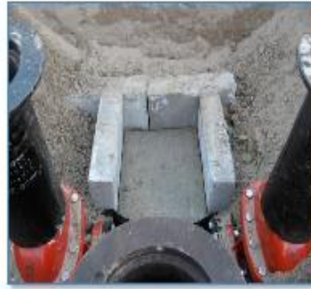
Hydrant Tee Ready for Thrust Protection
