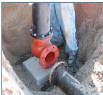
Hydrant Flanged to Protect from Separation
