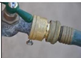
*Install vacuum breakers at hose bibs without anti-siphon devices.*
