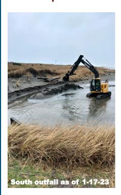
Are you wondering why the canal and Seabreeze Lake water levels are so high? All the recent storms pushed large amounts of debris (sand, logs, vegetation) toward the shore and the outfall gates become blocked. The south outfall is located at 328th and G Street and the north outfall is located at 350th and G Street. Pacific County was at both outfalls several times over the last
