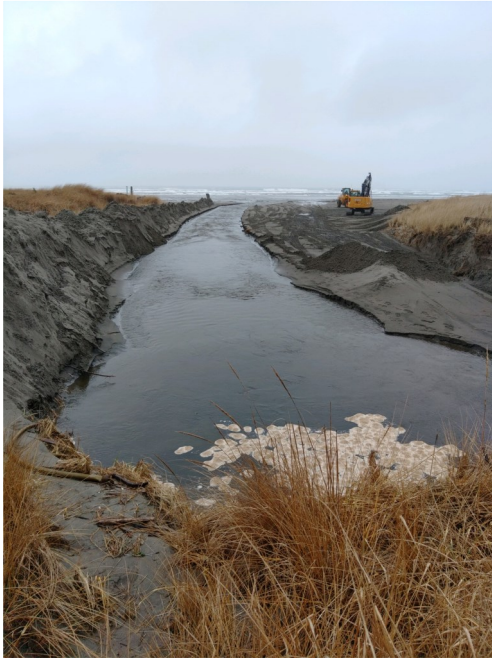
South Outfall during cleanout
